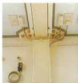
連棟部入電側
